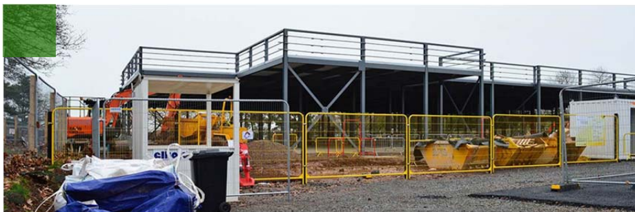
Work starts on the new OCC at Hindlip – October 2016
